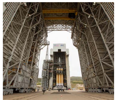
Mobile Assembly Shelter (MAS) Retraction: Delta IV NROL-82 PHOTO CREDIT: UNITED LAUNCH ALLIANCE
